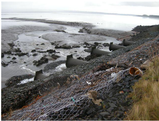
Figure 4: Pipes through embankment from lagoon to Forth
