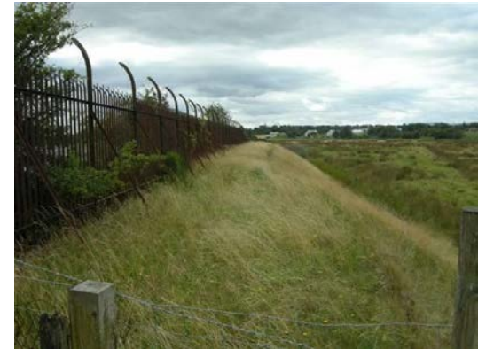
Figure 3 Palisade fence on top of embankment
