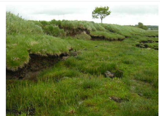
Figure 5: Southern embankment showing evidence of erosion May 2011
