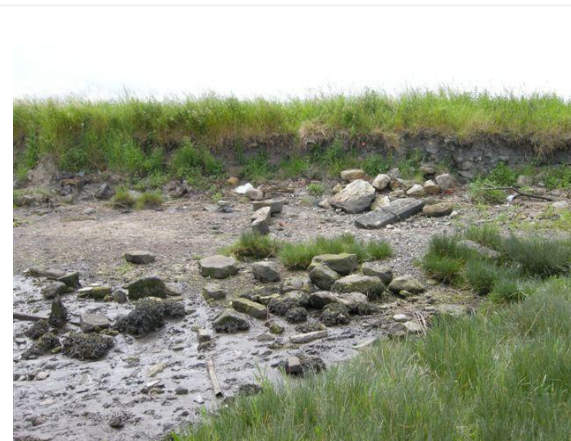
Figure 3: Eroding embankment on seaward side of embankment near sewage treatment works
