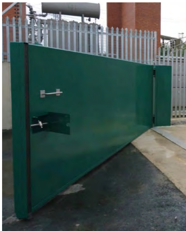
Example of a flood gate
