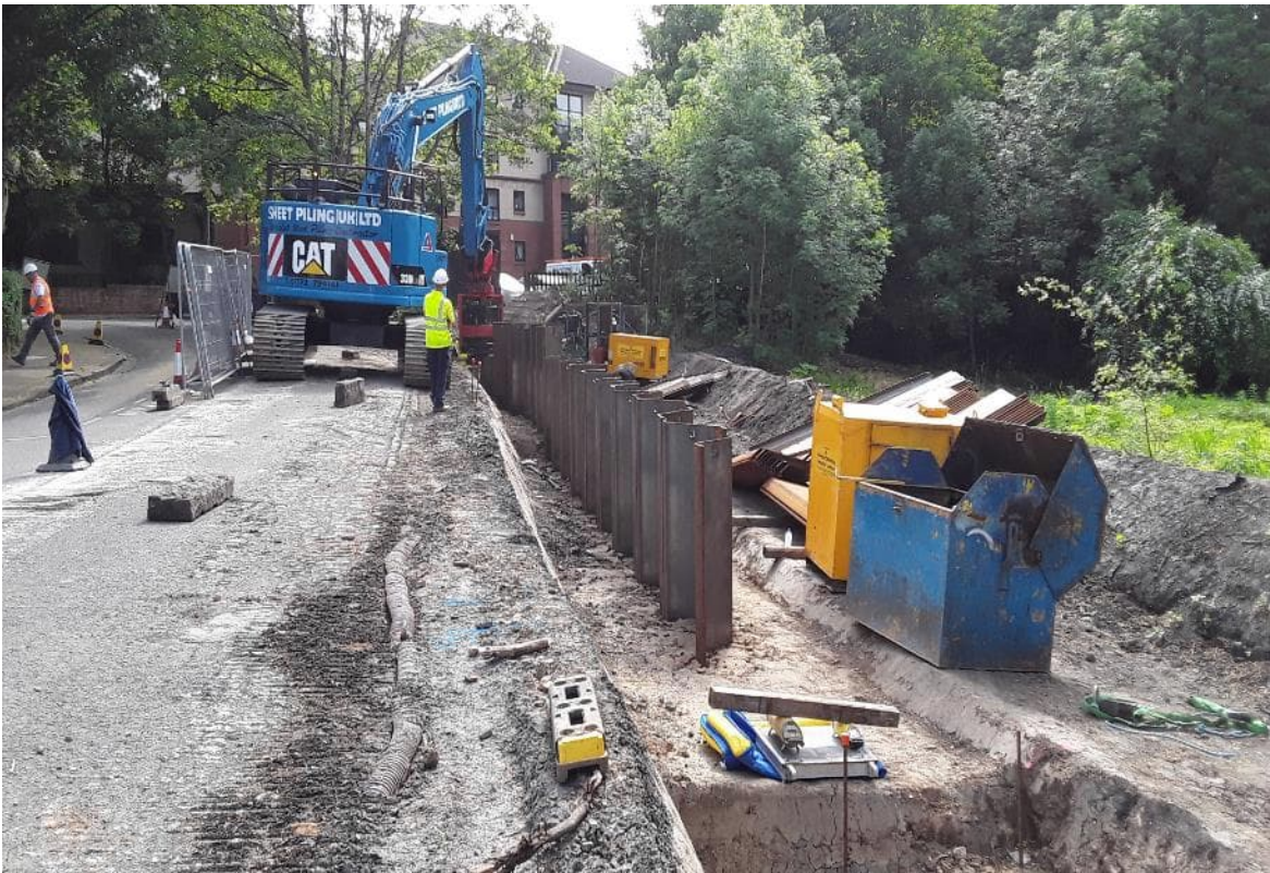
Figure 9 - White Cart Water FPS Phase 3 - Sheet piles being installed adjacent to road with Movax rig
