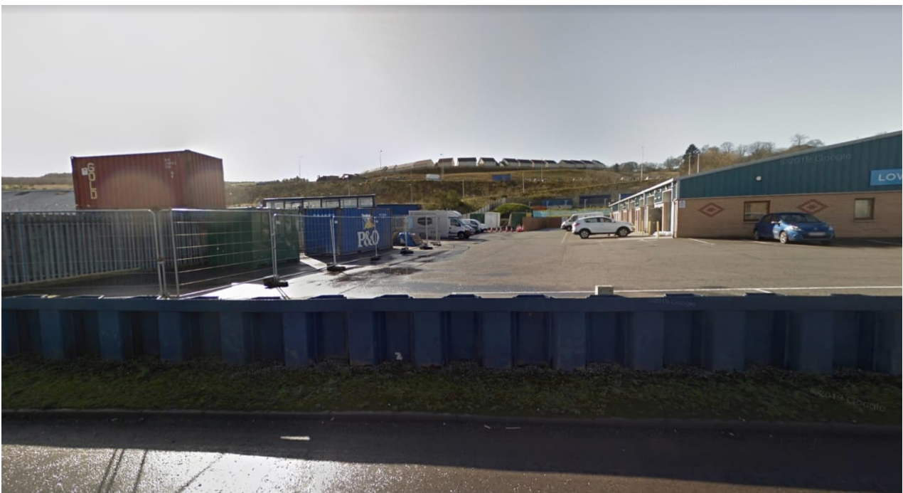
Figure 10 - Perth FPS – Steel Capping Plate/ Exposed Sheet Pile Flood Defence
