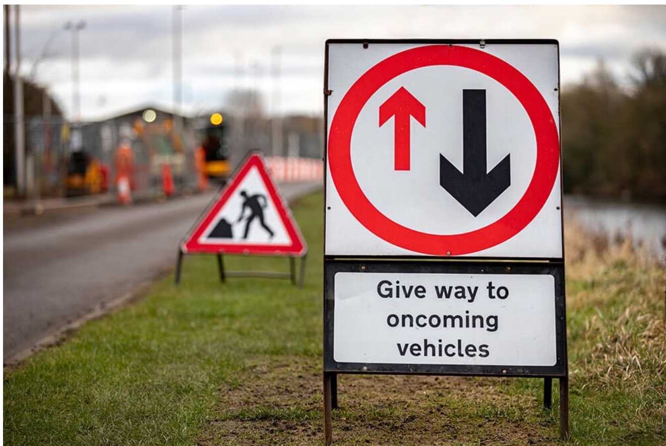
Figure 3 - Hawick Flood Protection Scheme Traffic Management – single lane closure
