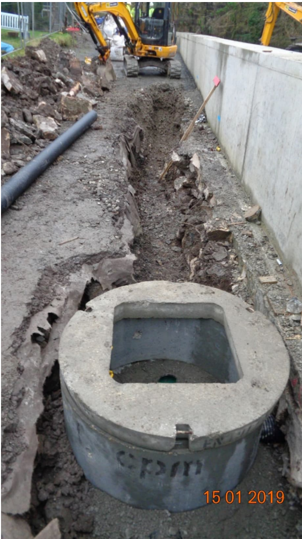
Figure 16 – White Cart Water FPS Phase 3 – Secondary Drainage Installation
