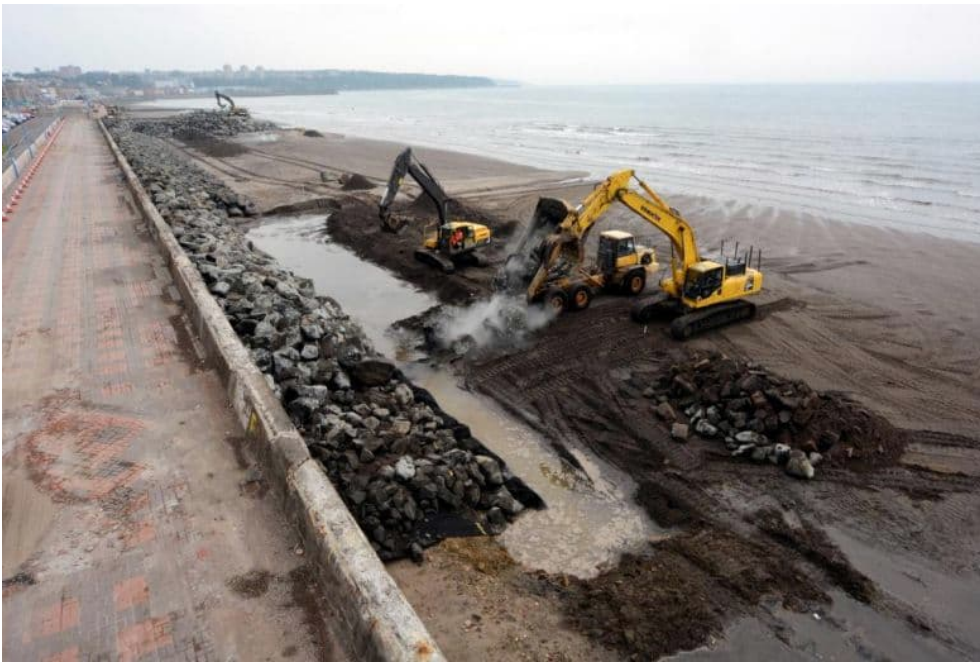
Figure 15 – Kirkcaldy Sea Wall – Rock Revetment Construction. Photo Courtesy VolerWessels UK
