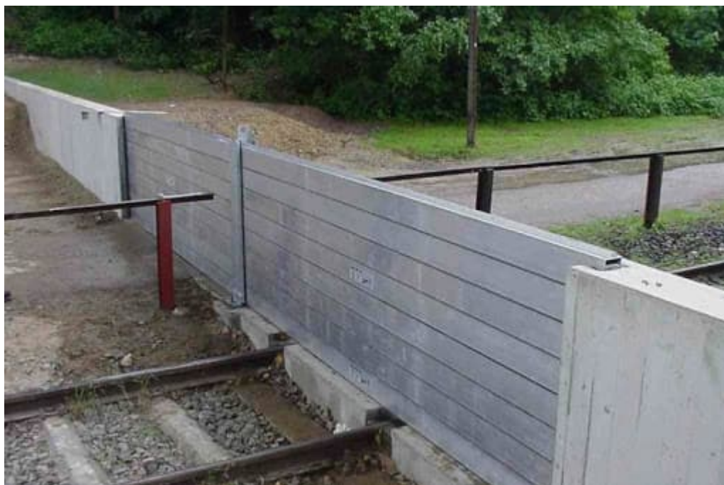
Figure 12 - Demountable Defence Across Rail Track
