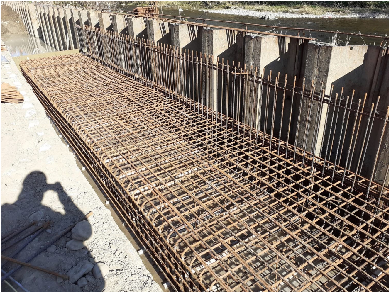
Figure 14 - Hawick FPS – In-situ Reinforced Concrete Wall Showing Base Reinforcement within Sheet Pile Cofferdam
