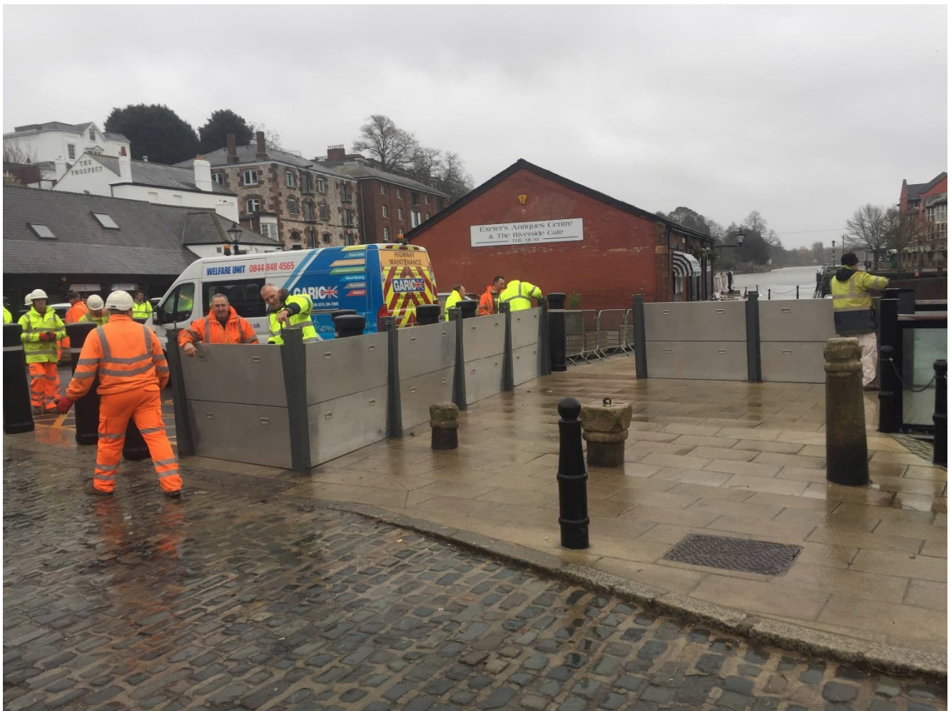
Figure 11 - Exeter FPS – Erection of Demountable Flood Defences
