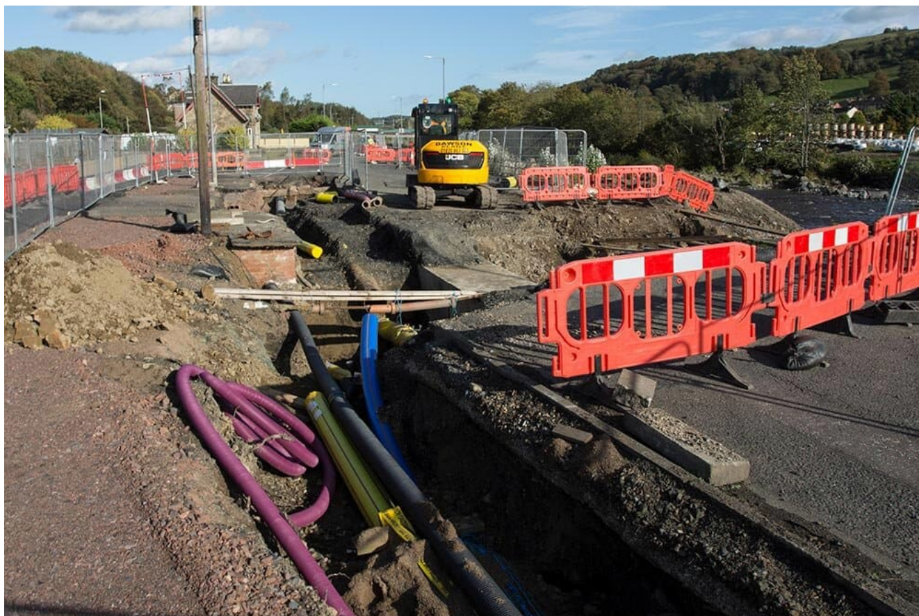
Figure 2 - Hawick Flood Protection Scheme Utility Diversions in Progress
