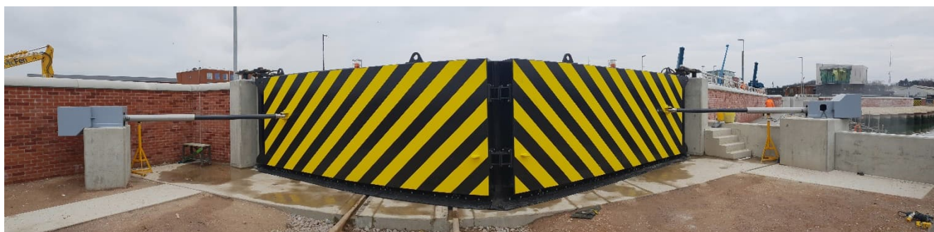
Figure 13 - Ipswich FPS – Flood Gate Across Rail Track
