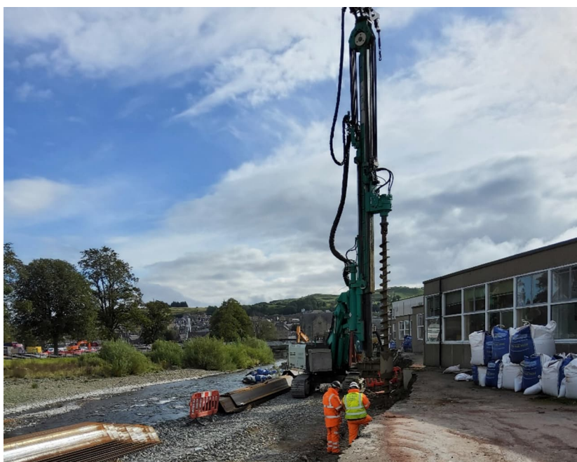
Figure 8 – Hawick FPS – Pre-augering ahead of pile installation
