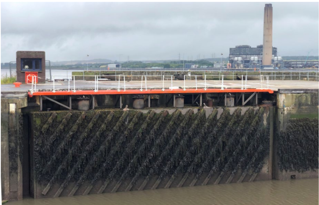
Figure 5: view of western leaf of outer lock gate in its open position
