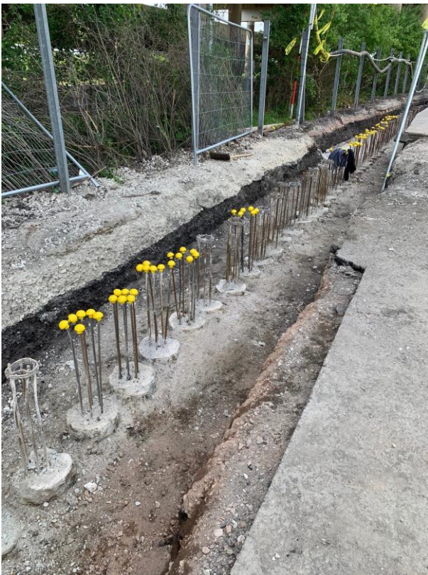
Figure 7, Bromford Flood Risk Management Scheme – Secant pile wall ready for reinforced concrete stem to be constructed.
