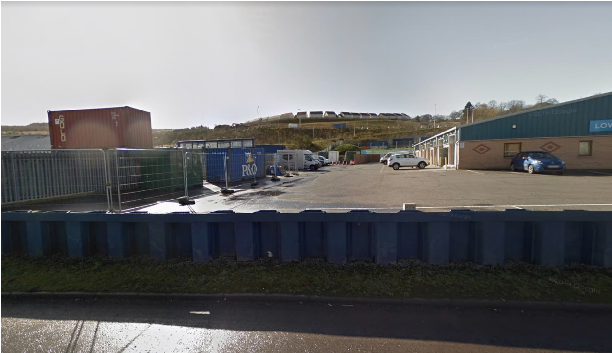
Figure 3 – Coated exposed sheet pile floodwall (Perth Flood Prevention Scheme)
