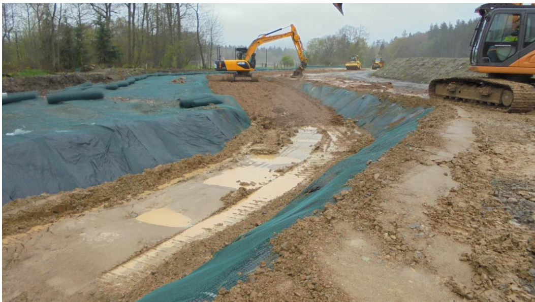
Figure 4, Earth embankment cut-off trench (Selkirk FPS)
