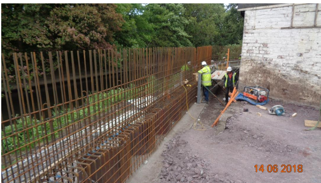
Figure 6, Sheet pile with reinforced concrete stem (White Cart Water FPS)
