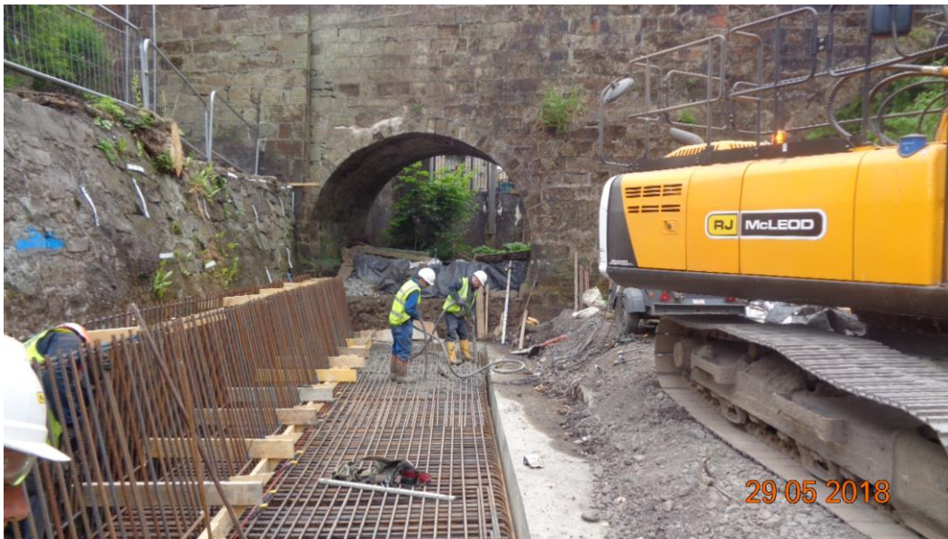
Figure 8, Reinforced concrete cantilever wall (White Cart Water FPS)
