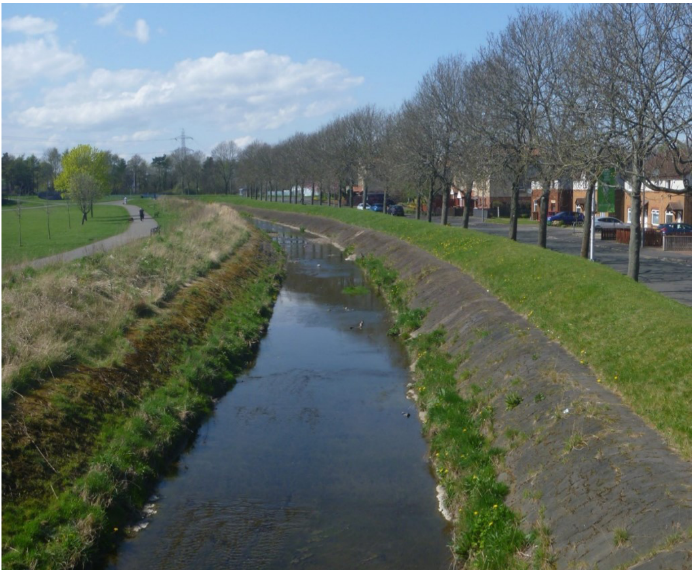
Grangemouth's Flood Relief Channel.
