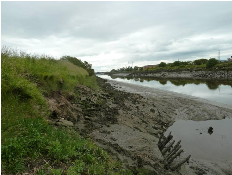
Plate 12. Erosion of the seawall dividing the River Carron and the site, around the inlet pipe.
