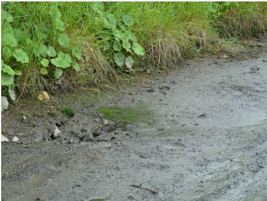
Plate 13. Signs of leaks through the seawall.
