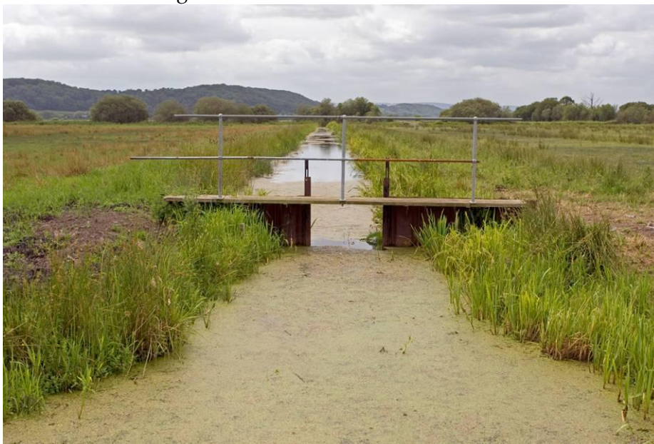
Plate 2. An example of a simple drop board sluice, which could be installed at the inlet ditch to control water levels in the lagoons.
