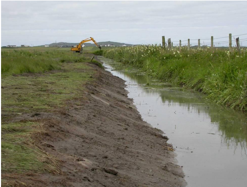
Plate 3. Example of ditch reprofiling at RSPB Scotland's Reef reserve.
