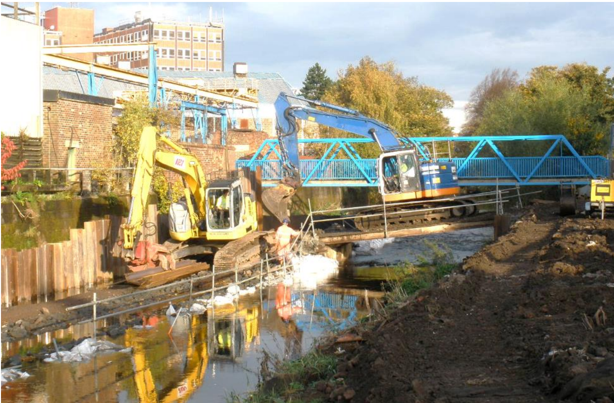
Figure 4: Example of a Bailey bridge in use
